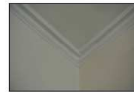
Existing plaster cornice
