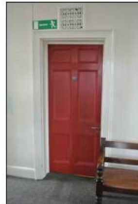
Existing door adjacent to new opening
